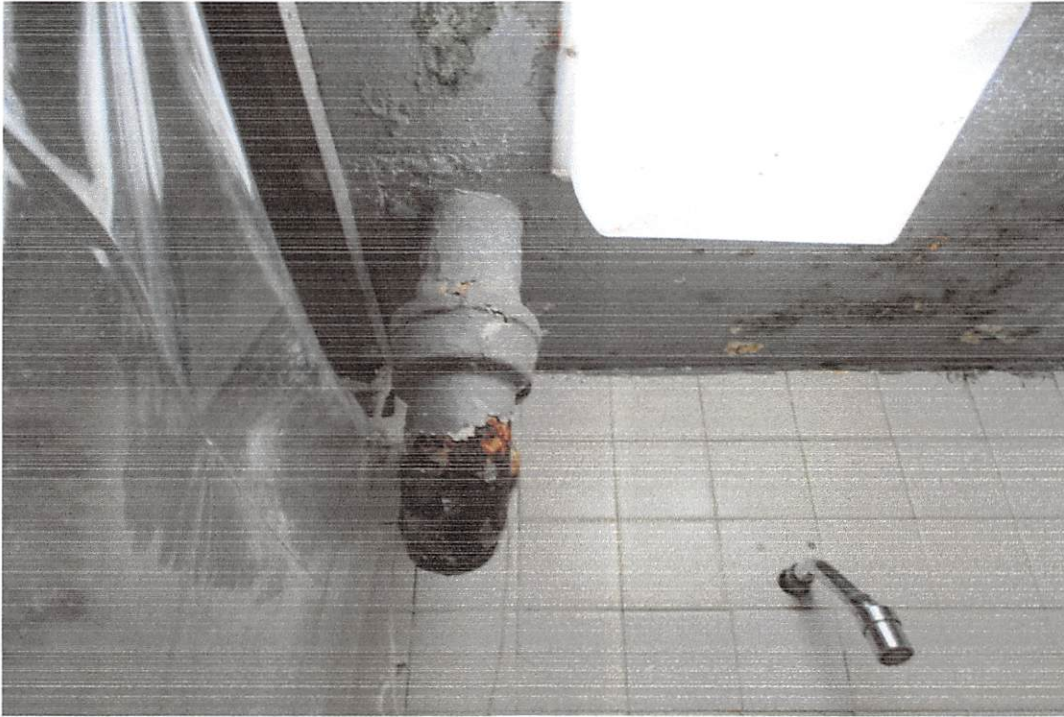
Photograph #13 Discoloration and water damage
